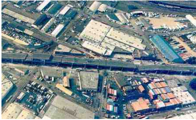
1 / The collapsed section of the Nimitz Freeway
